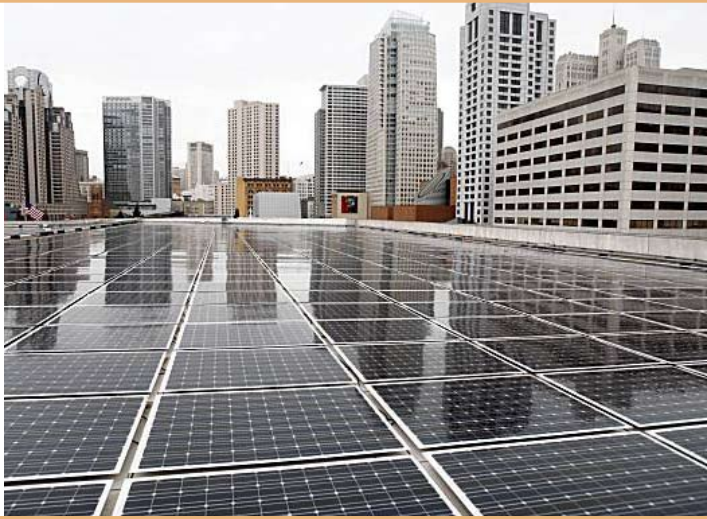
A 675-kilowatt flat roof solar PV system on the Moscone Convention Center in San Francisco, California.
