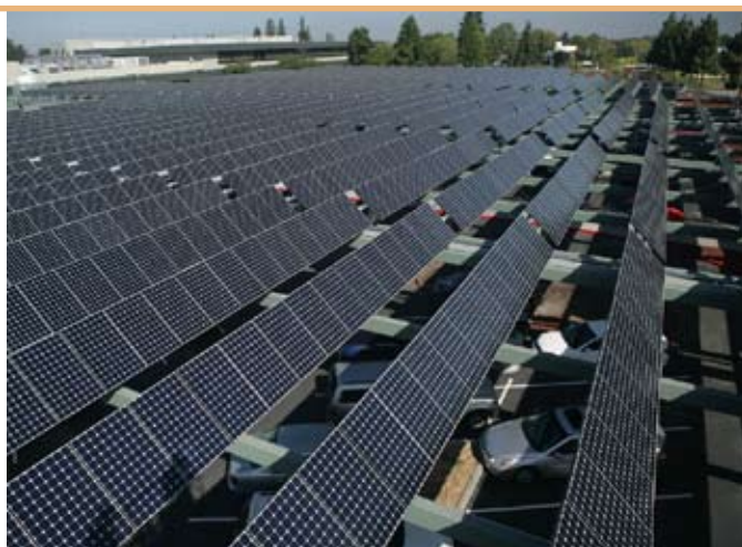
A 2-megawatt solar PV system, one of the largest corporate solar power installations in the U.S., covers the Applied Materials parking lot in Sunnyvale, California. The 8,000 panels change their tilt to track the sun’s position.
