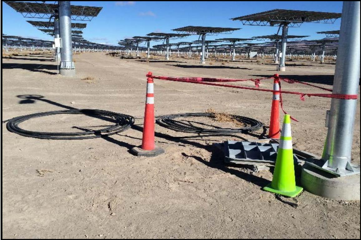
Figure 7 – Electrical conductor lying in spools ready to be pulled into conduit via a manhole.
